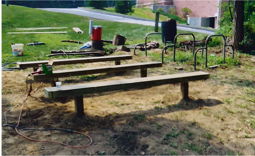
↑ Benches under construction with picnic table frame in backdrop
