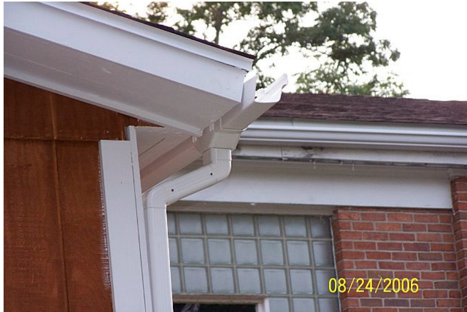
Gutters and soffits placed on new shed
