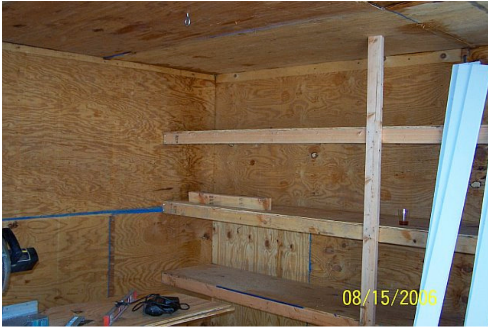
Shelves being built
