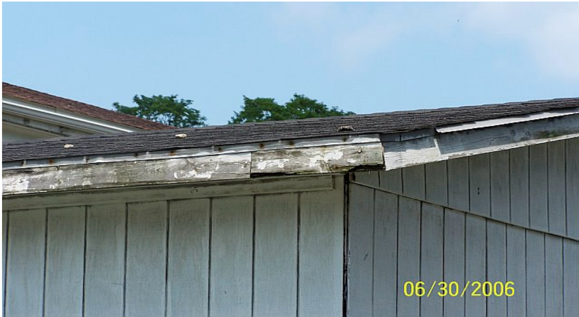
Picture of the soffits and roof of the old shed
