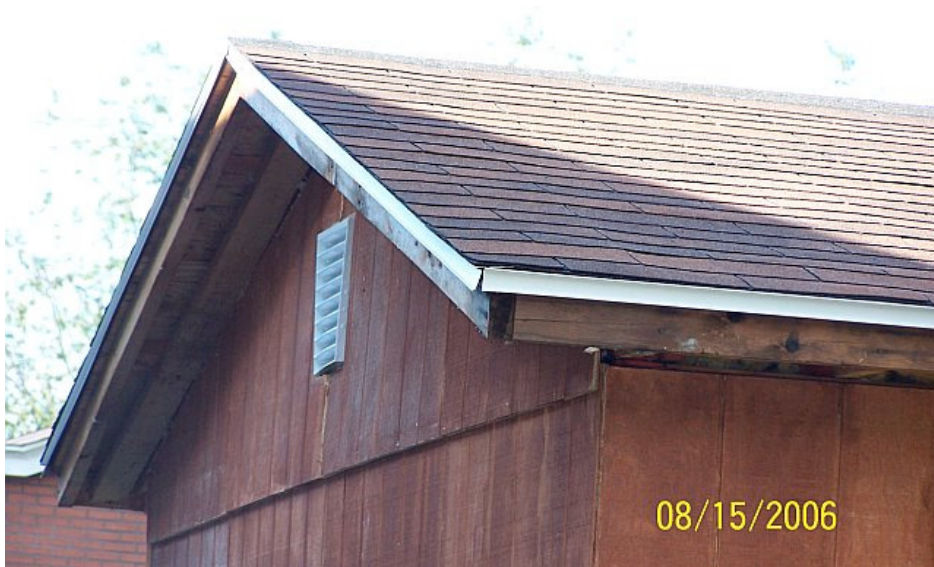
Shingles placed on roof along with T111 nailed up
